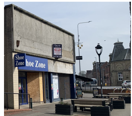
A boarded-up empty shop in Goole, which could become a pilot HSRA project.
