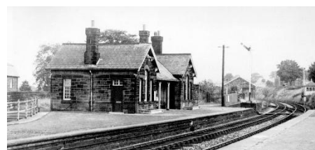
1920s view of the station looking towards Ilkley, showing location of signal box
